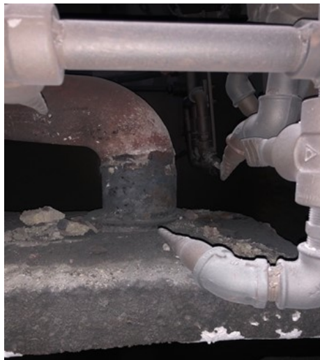
Figure 12. Additional air-blowing nozzles for removal of residuals.
